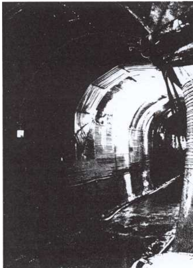
Fig. 6 Instrument tubes in the grouting gallery
