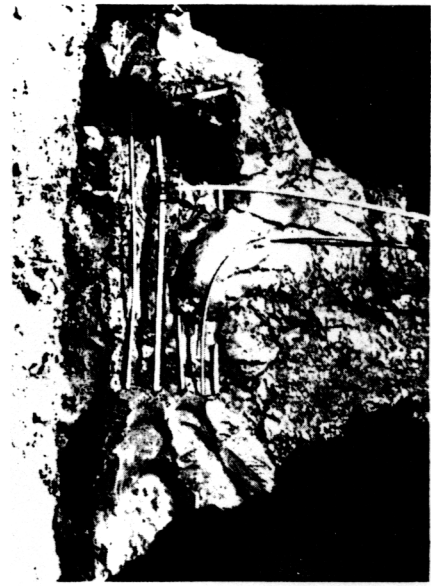
Fig. 7 Arrangement of the transmission tube line in a ditch in the dam fill. Fixing the tubing line sections by clay packing
